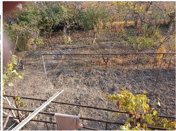
The unfinished greenhouse
