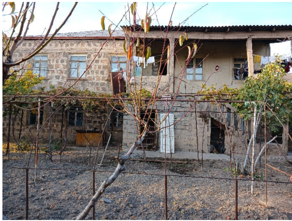
The house and part of the greenhouse.
